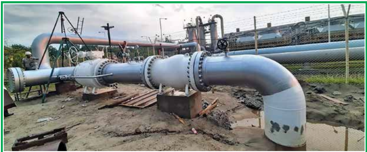
Modification activities at Ashuganj Gas Compressor Station
