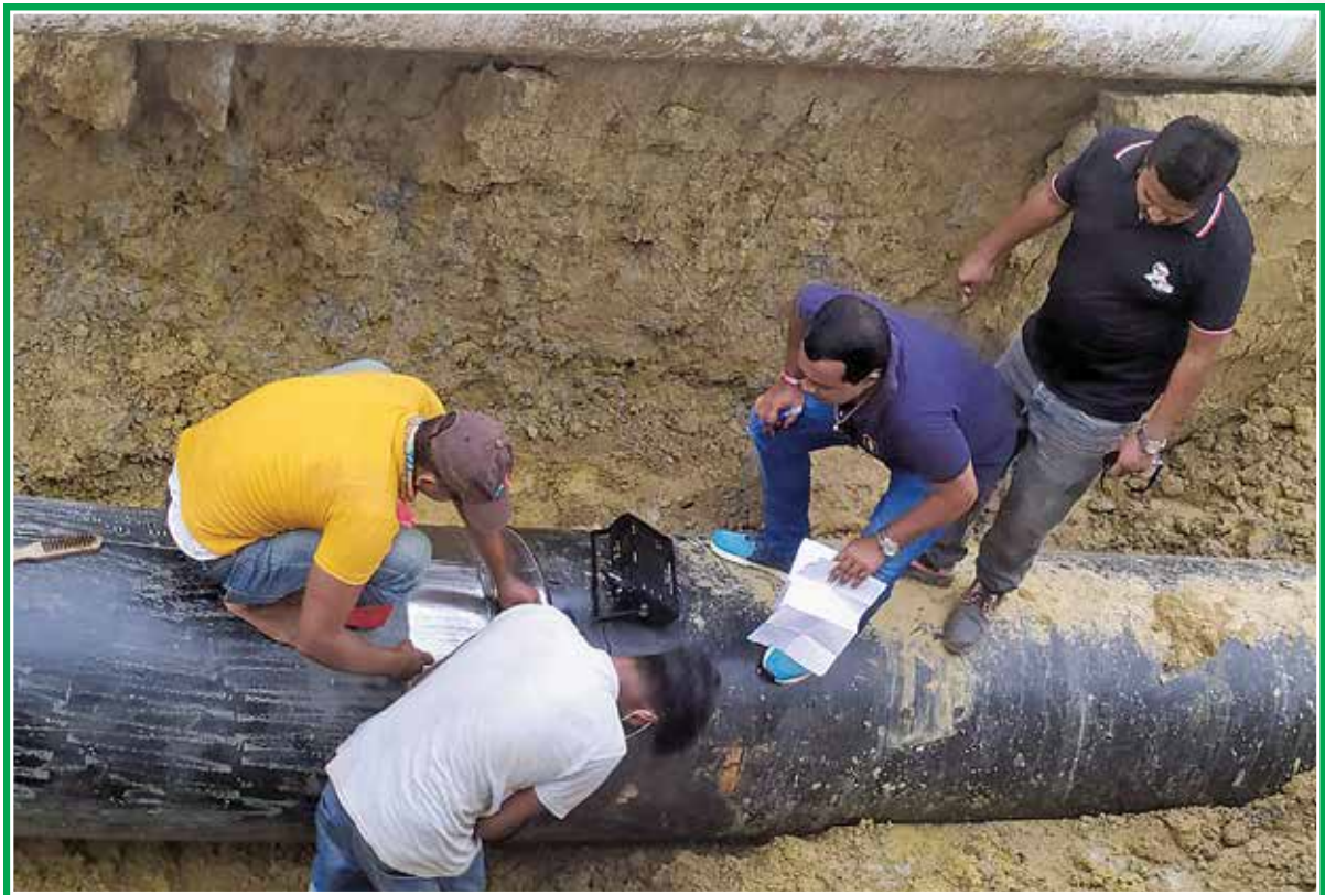
30" dia Dhanua-Elenga Pipeline Crossing underneath 24" dia B-B pipeline
