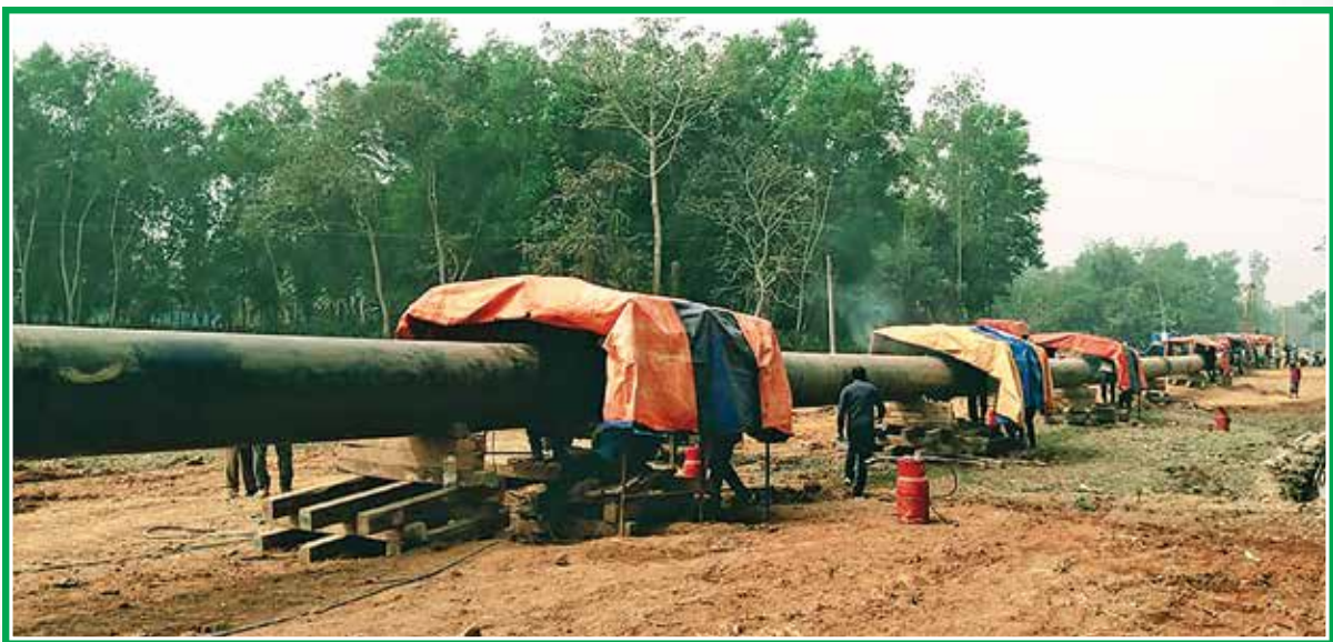
Welding Works of 30" dia linepipes under Dhanua-Nalka Project
