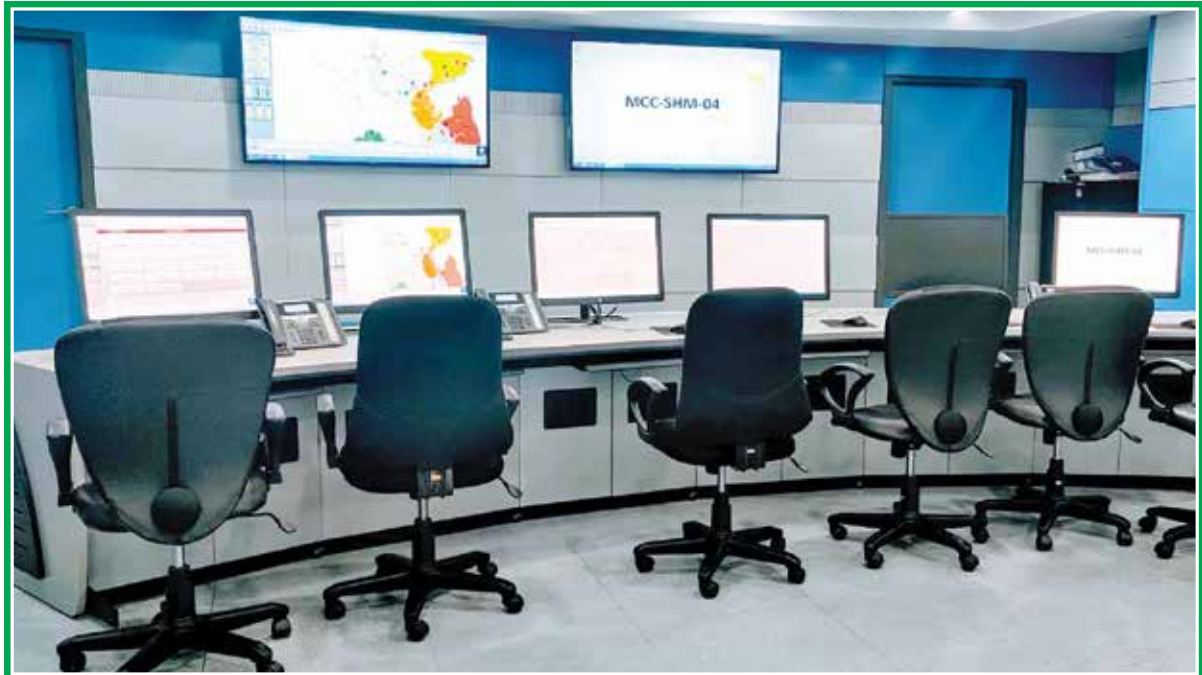
Master Control Center of SCADA System at GTCL Head Office
