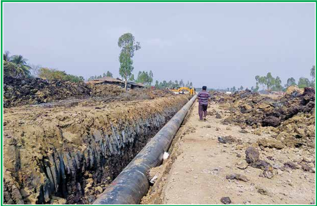
Laying of 42" dia Pipeline under Moheshkhali-Anowara Parallel Pipeline Project
